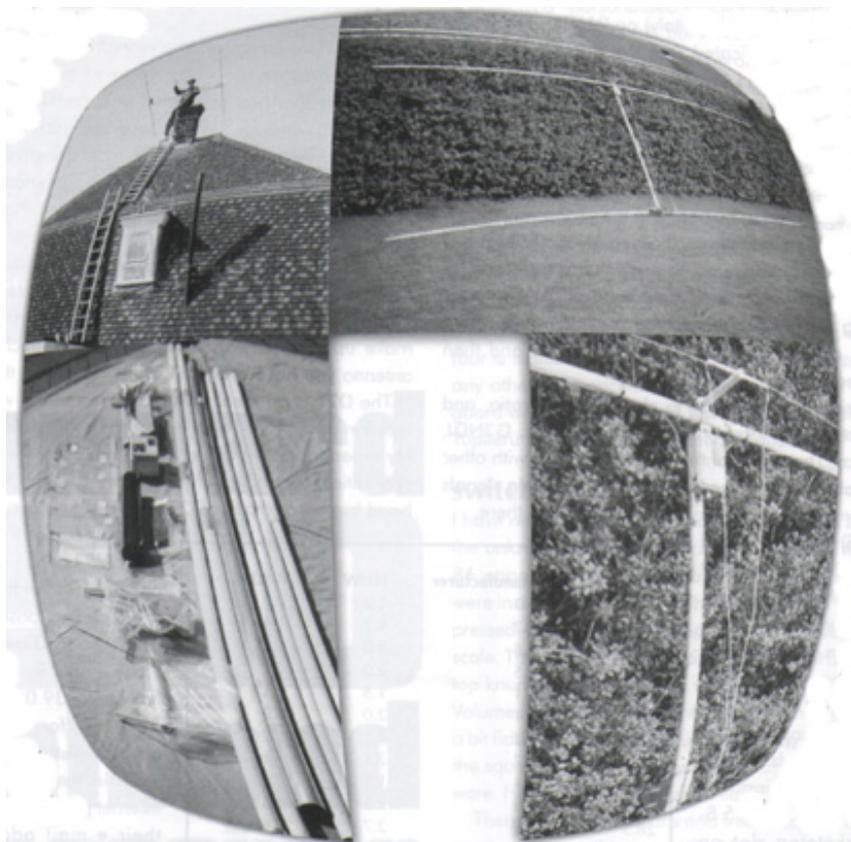
( Clockwise from bottom left ) : The kit of parts for the D2T antenna. All the small parts, including all the nuts and bolts are enclosed in polythene bags, carefully labelled with a 13-digit part number ; Fixing the antenna ready for testing. The antenna is mounted on a short mast on a KR-600RC rotator, which is fixed to the chimney using a double clamp ; The completed D2T antenna ; Close-up showing construction details
